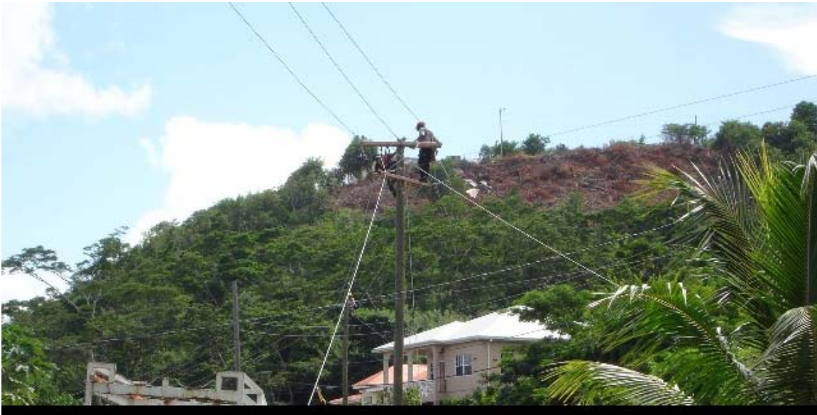
Grenlec installs poles at site this week
